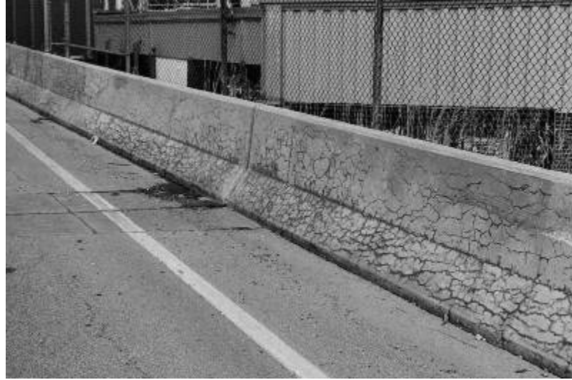
Figure 1-6: Bridge parapet showing ASR cracking [72]
