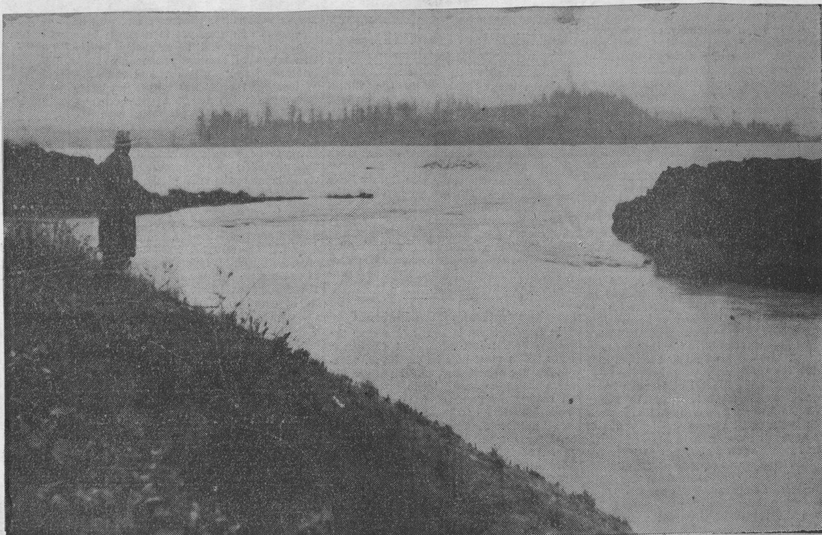
WHERE DIKE LET GO. Wapato lake, at Gaston, last night was inundated as of old, after flood waters dug a 60-foot hole through the $75,000 dike, intended to keep the lake bed dry. Shown in the foreground is the swollen moat outside the dike and the break in the wall. The flooded area in the background was an onion field a few days ago. Flood stories on pages 1 and 4.
