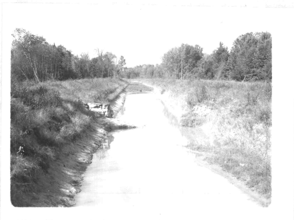
Figure 3. 1975 Cypress Creek drainage channel located 8.5 kilometers from mouth.
