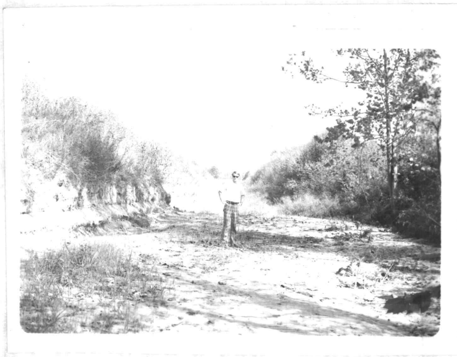
Figure 4. 1975 Cypress Creek drainage channel located 10.6 kilometers from mouth.
