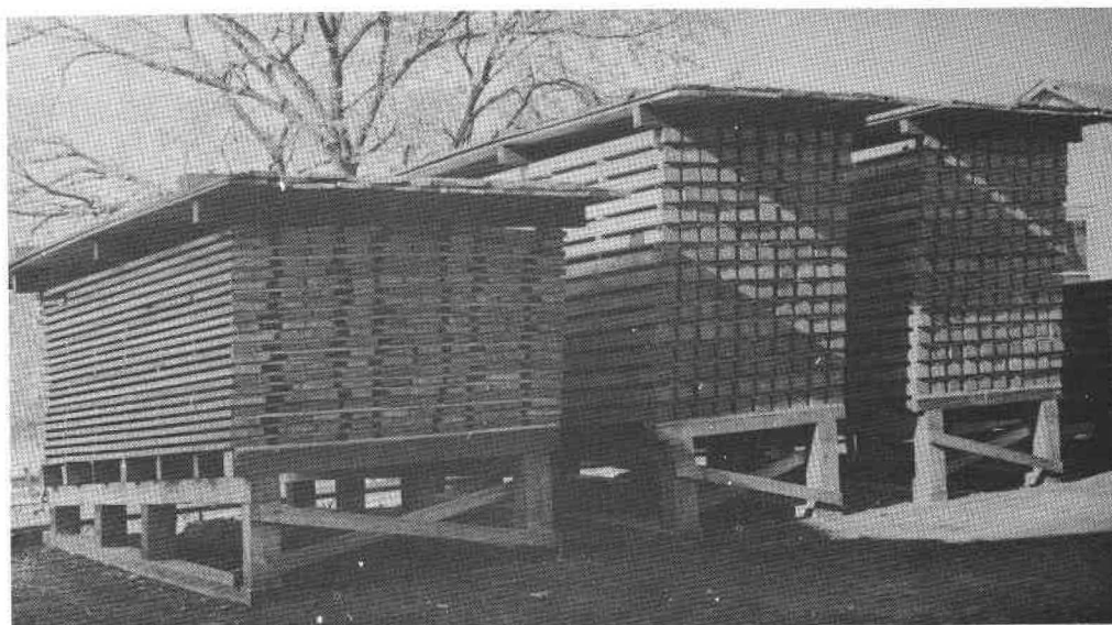
Figure 20. -- When the piers of relatively narrow pile foundations do not extend into the ground, they should be braced to prevent lateral tipping. These experimental piles illustrate most of the features of good air-seasoning practice.
