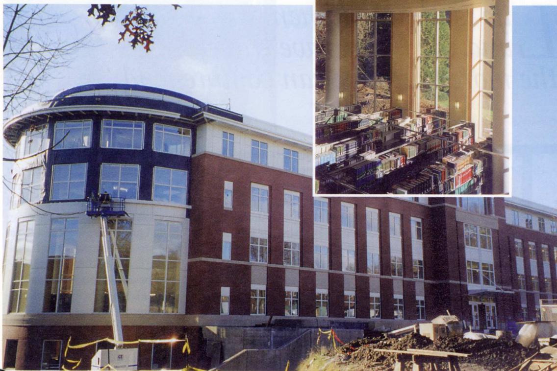
Left: Window trim being applied to rotunda
