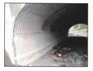
Figure 8. Mud lines as seen in the US97 culvert indicating the height of wave crests during the 1997 Whitney Creek debris flow.
