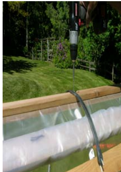
Figure 12. Attach the bungee cord at its center to the backbone. This will hold the rolled-up plastic for easy access to both sides of the raised-bed cloche.
