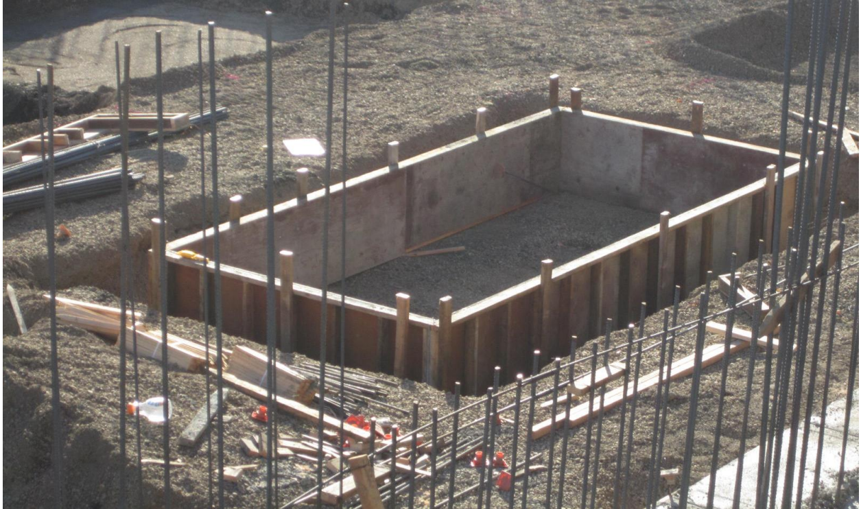
Figure 4.7: Footing Foundation, Project 2
