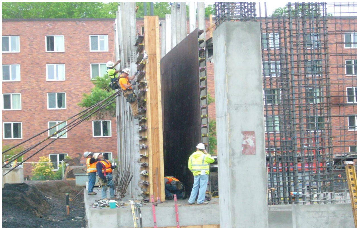
Figure 4.2: Wall forms being Erected, Project 1
