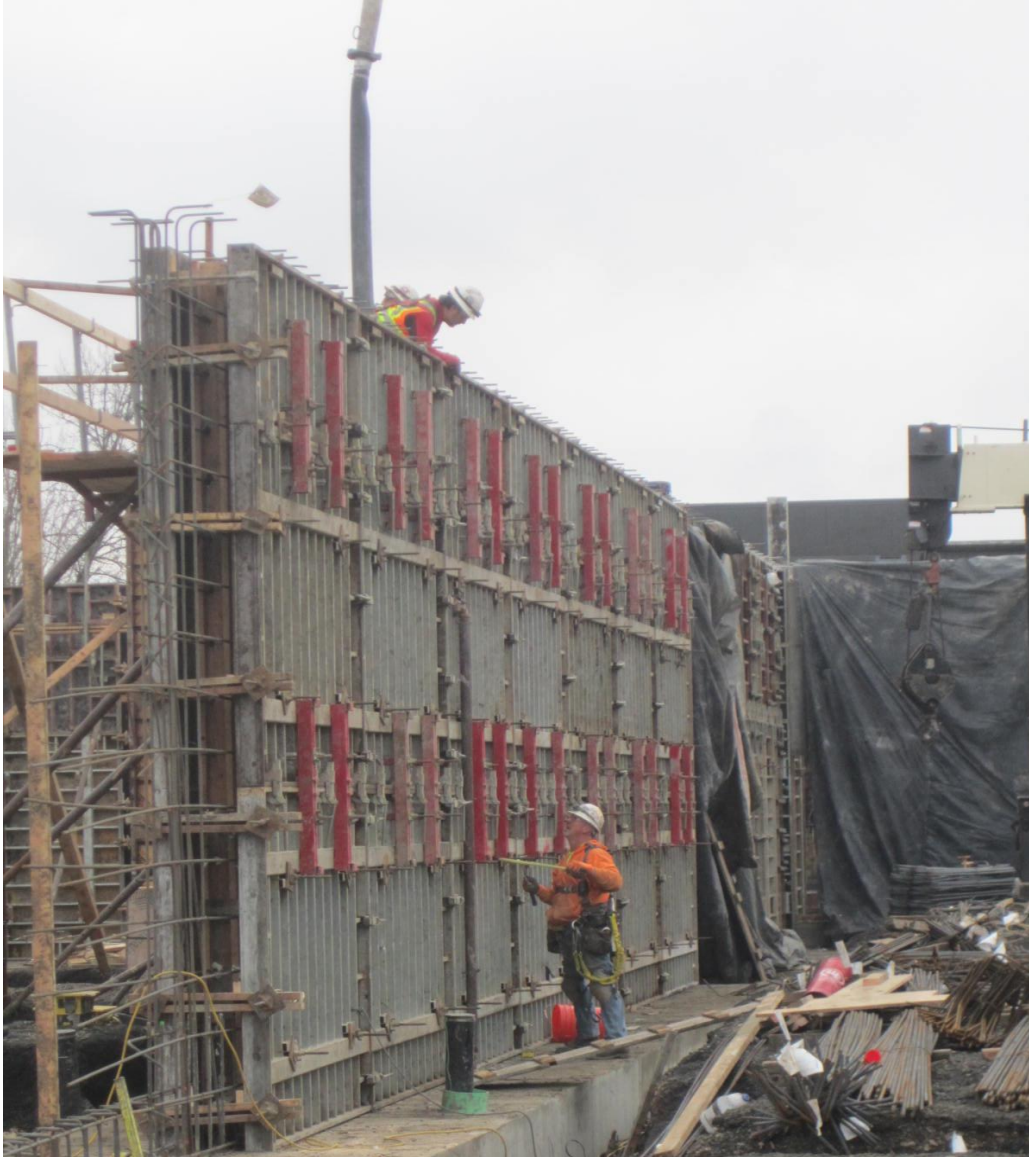
Figure 4.9: Wall Formwork, Project 3
