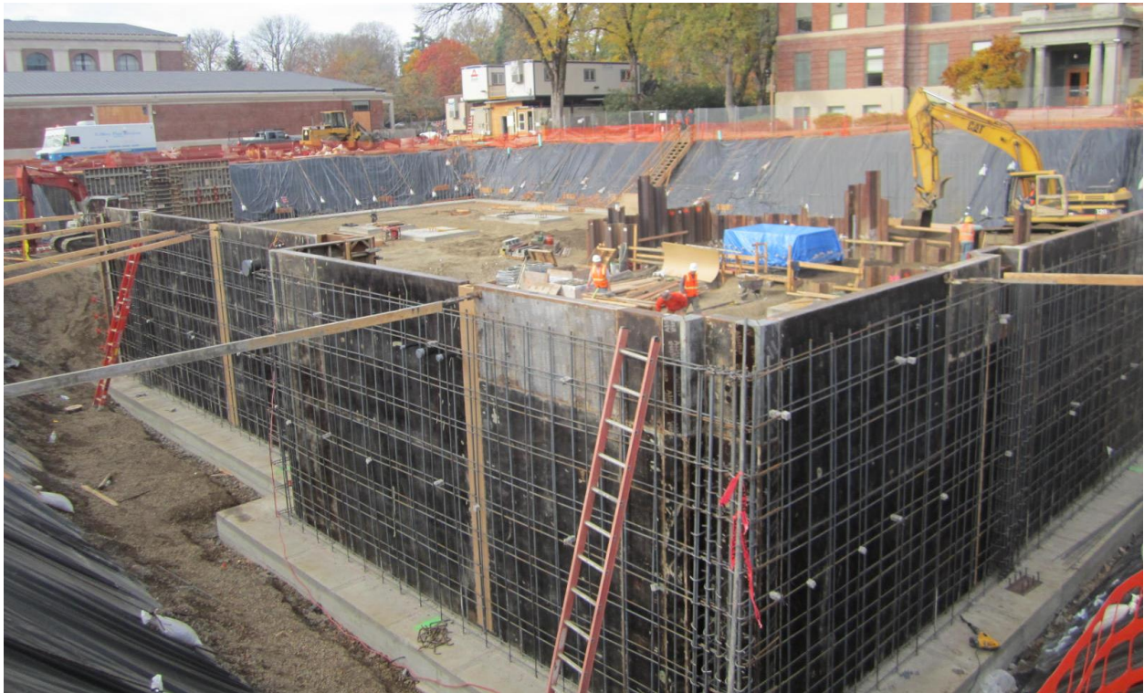
Figure 4.5: Wall formwork systems partially erected, Project 2
