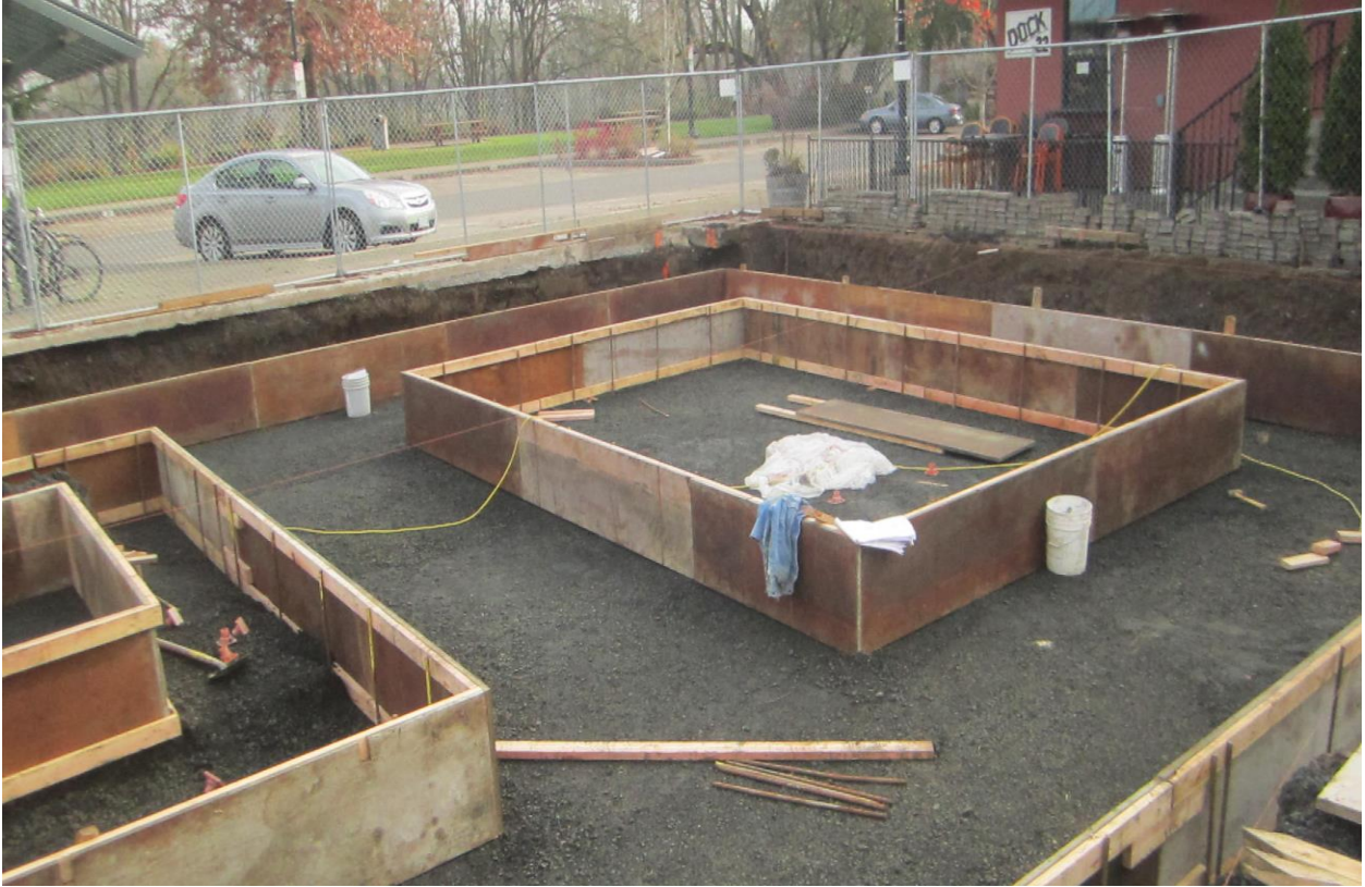
Figure 4.8: Footing Formwork, Project 3
