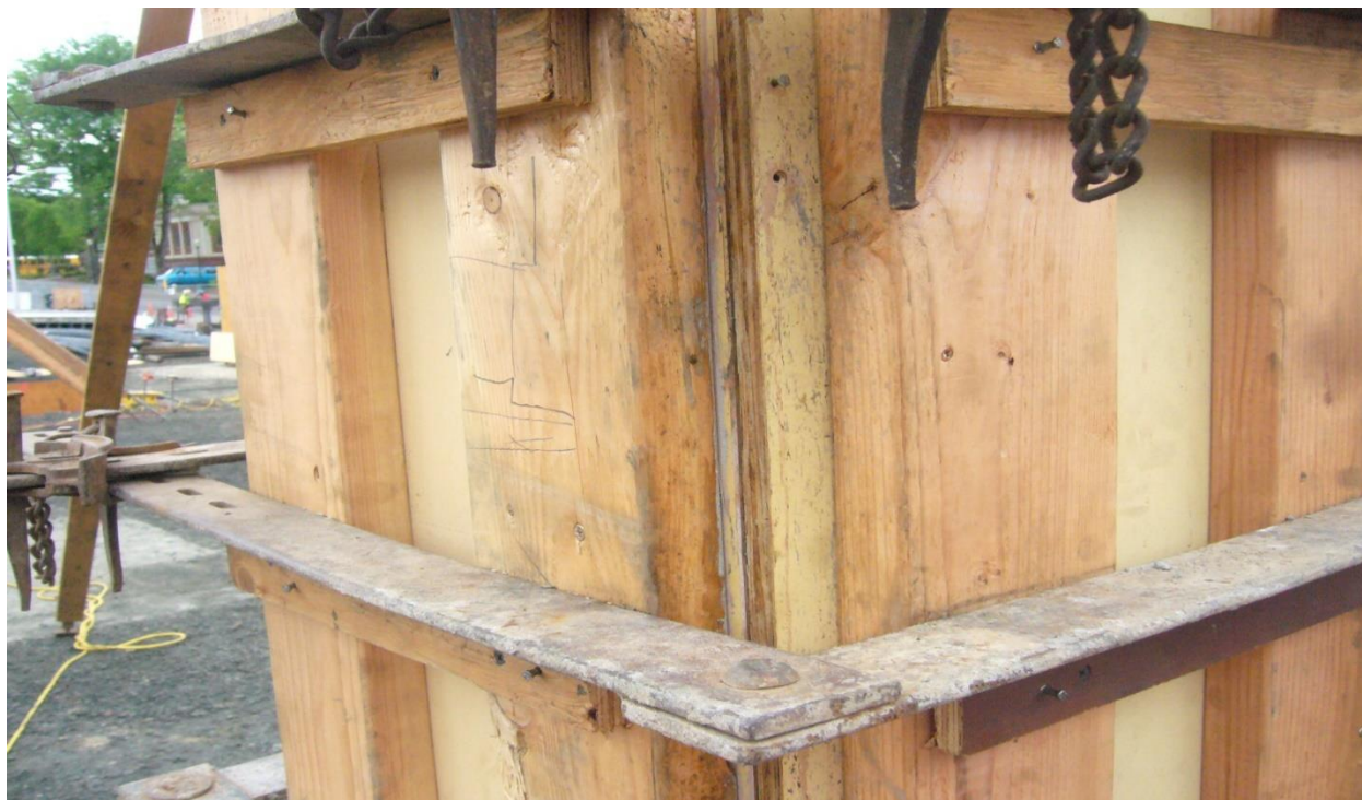
Figure 4.3: Erected column form, Project 1
