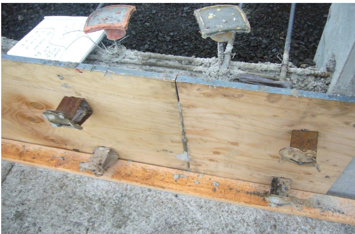
Figure 4.4: Base wall formwork ready to be stripped, Project 1
