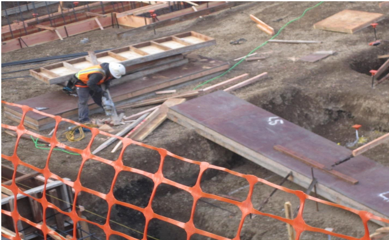
Figure 4.6: Preparation of formwork components, Project 2
