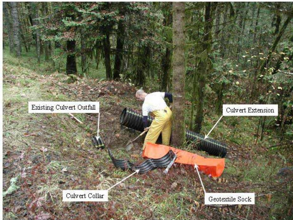
Figure 3. 5 The author preparing site for installation of sediment trap. The vinyl membrane is not pictured. Roadway is left of the picture.
