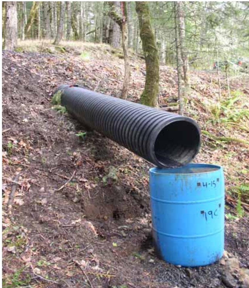
Figure 3. 6 Barrel + sock sediment trap as used at culverts 30, 66, 76, 81, 88, and 98. Geotextile sock is extended inside barrel but not in view in this picture.
