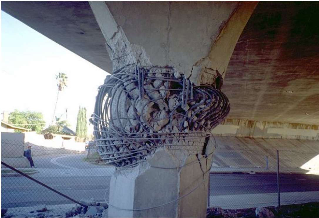
Figure 1.1: Failed bridge column due to the 1994 Northridge, California shallow, crustal earthquake (ACE-MRL, 2013).
