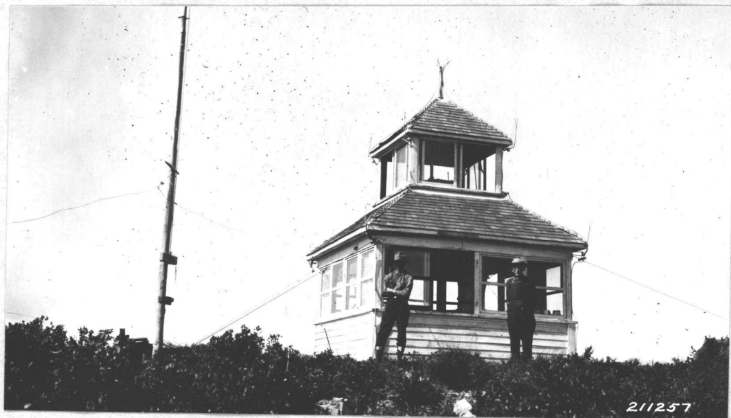
An adequate lookout house, comprising living quarters and observatory. Lookout can render efficient services by not being exposed to elements. Protection from lightning is given through cables and lightning rods.
