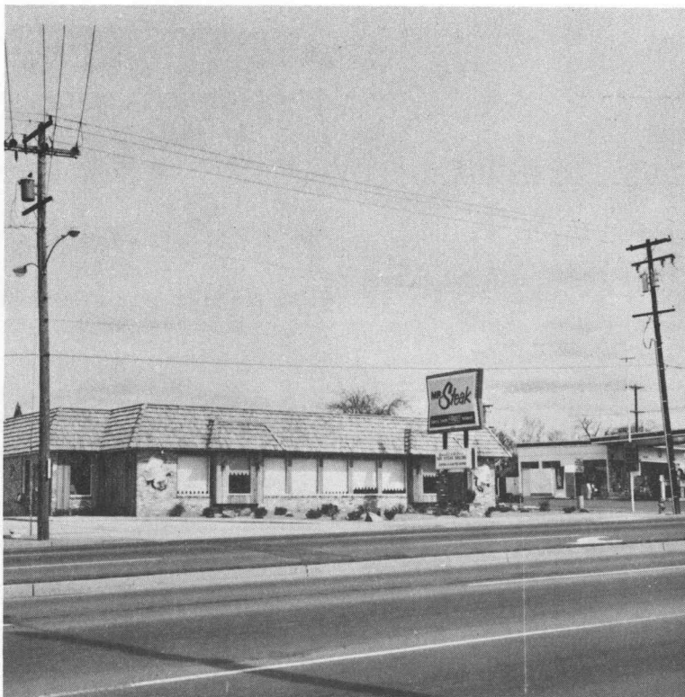
Mansard roof construction is popular in the Eugene area and uses lots of cedar shakes.
