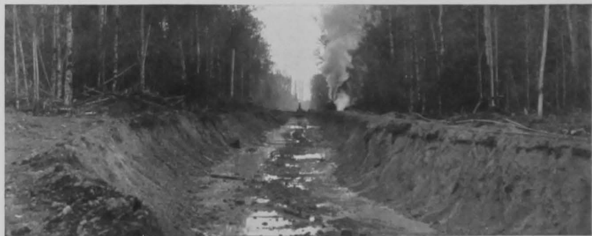
Cutting canal to divert White River into Lake Tapps.
