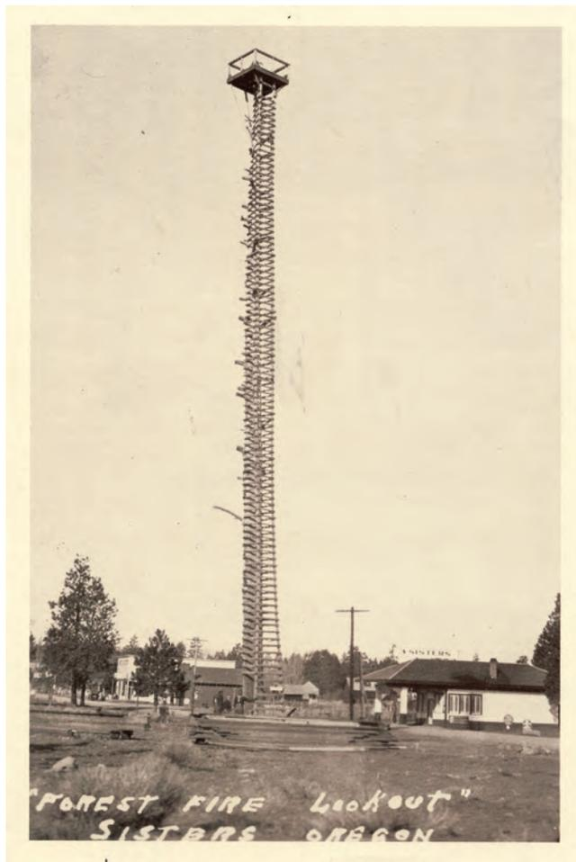
Figure 62. Fire tower in Sisters, Oregon circa 1925. The tower was constructed around a 110-foot-tall ponderosa pine.
