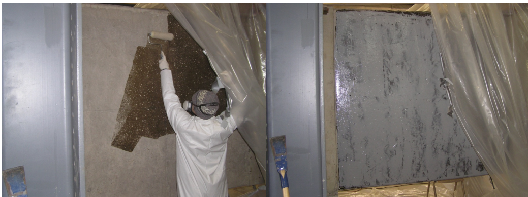
Fig. 3.48 – CFRP bent cap installation: primer (left) and putty (right).
