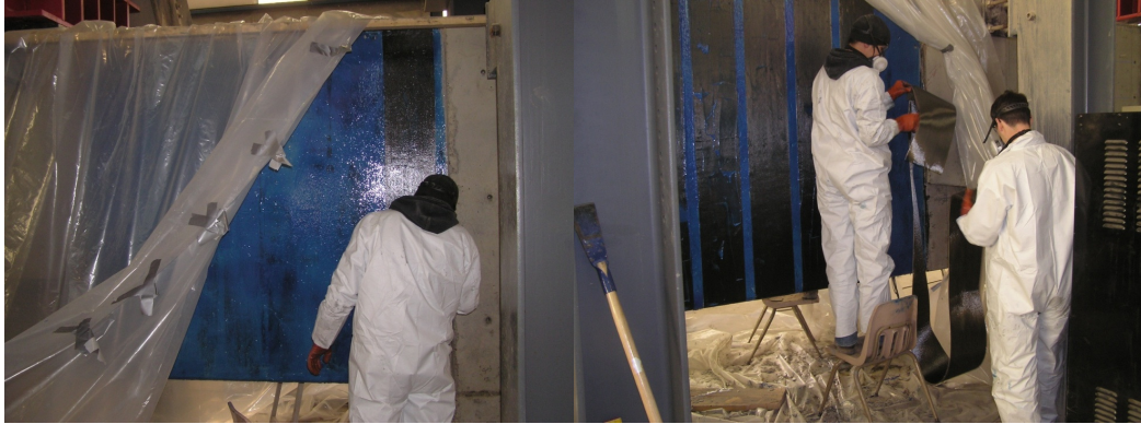
Fig. 3.49 – CFRP bent cap installation: strip installation.
