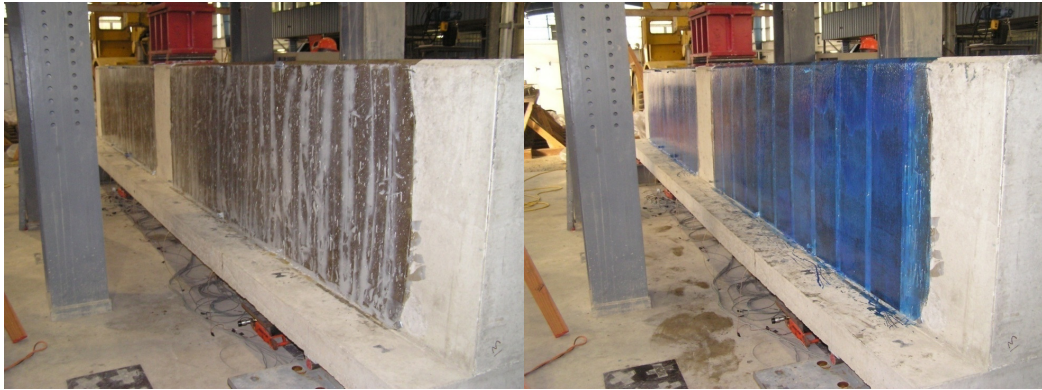
Fig. 3.44 – CFRP installation: putty installation (left) and FRP strips with saturant (right).
