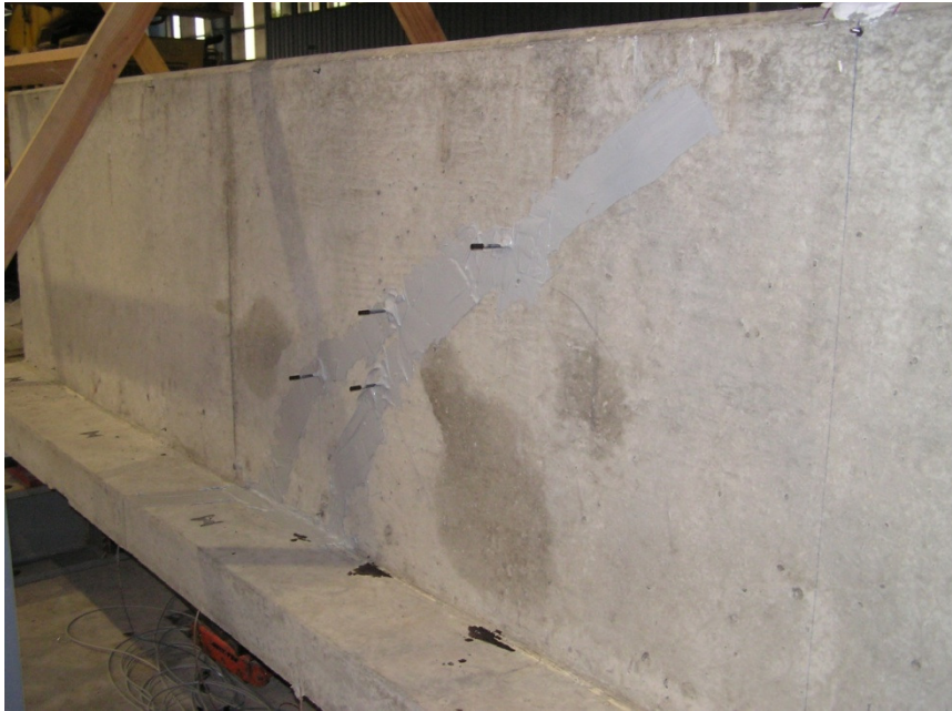
Fig. 3.42 – CFRP beam installation: epoxy injection.
