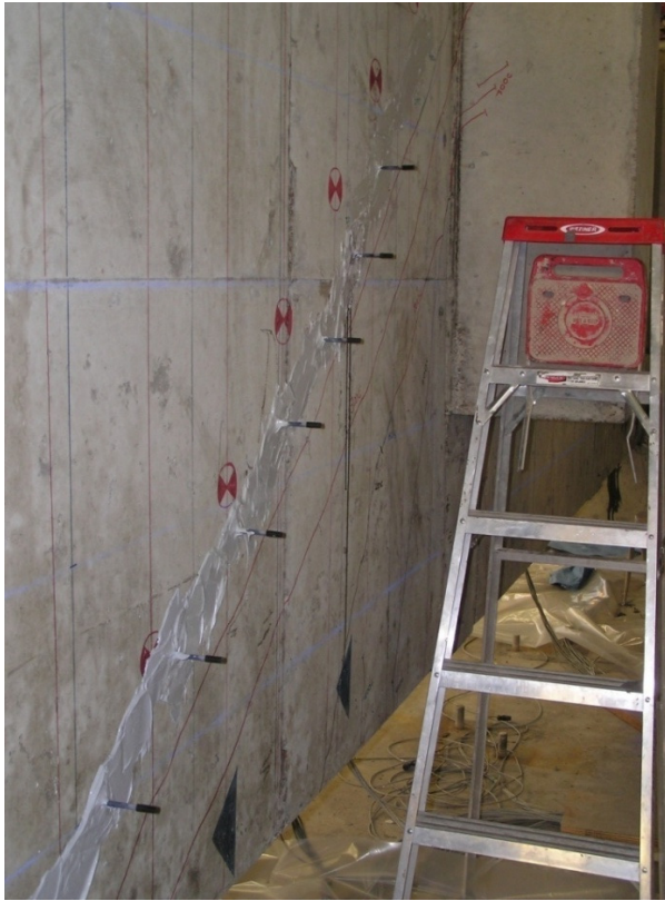
Fig. 3.47 – CFRP bent cap installation: epoxy injection.
