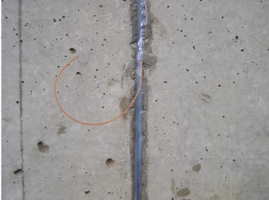
Fig. 3.46 – NSM installation: final product.
