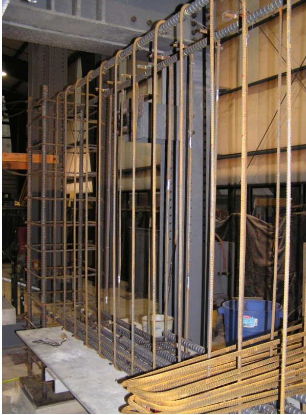
Fig. 3.35 – Typical bent cap stirrup assembly.
