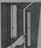
Fitted Interlocking Metal Channels (J-Strips)—Very difficult to install. Exceptionally good weather seal. Invisible when installed. Not exposed to possible damage.
