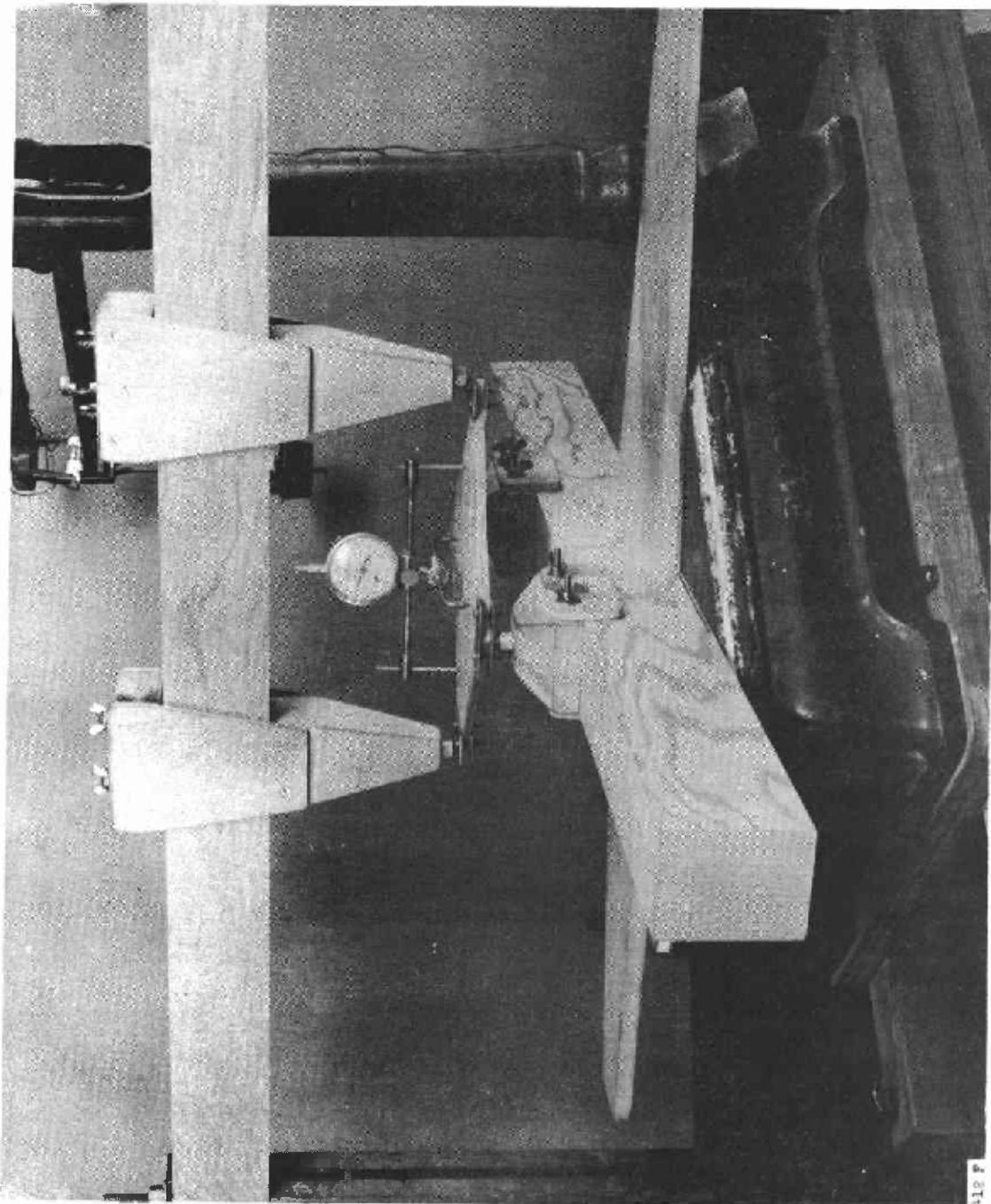
Figure 5.---Standard plate shear apparatus for measuring modulus of rigidity.
