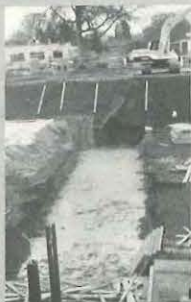
A sea of concrete. Construction workers pour footings for the new Laboratory.
