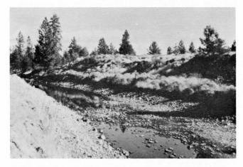
Figure 20. Canal at end of irrigation season (improperly screened or unscreened canals lead to considerable losses of brown trout).
