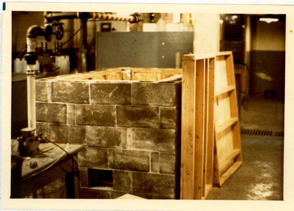
Figure 16. Photograph showing the cinder-block enclosure built around the compressor. Also shown are the plywood and 2 x 4 lids prior to being filled with sand.
