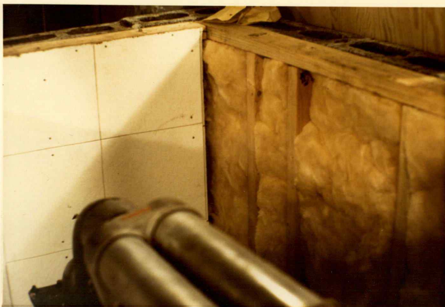
Figure 15. Photograph showing the glass fiber insulation and "accoustical" tile used to suppress the machinery noise of the compressor.
