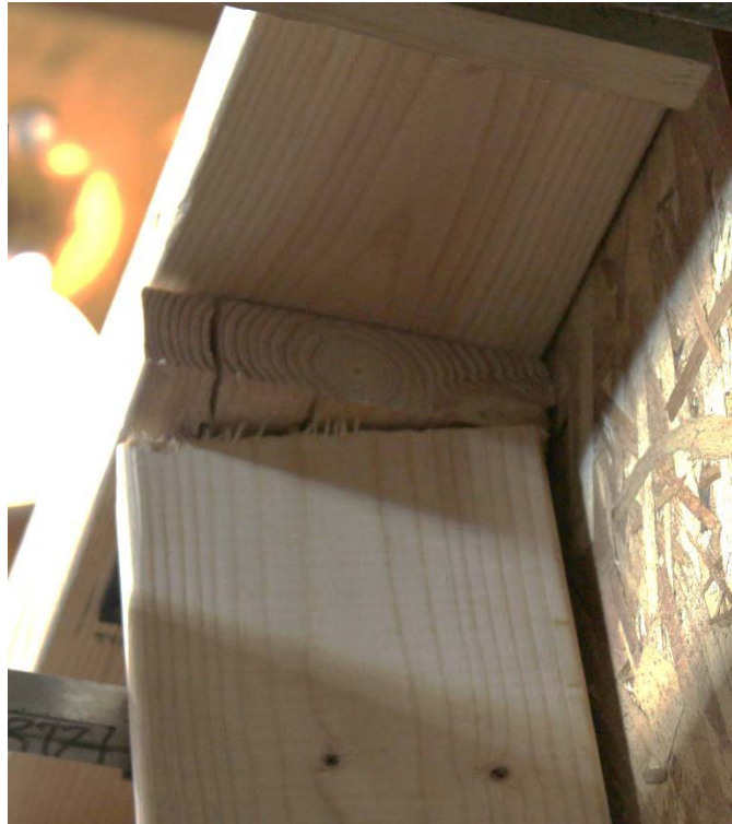
Fig. 2.10: Top plate splitting at stud connection
