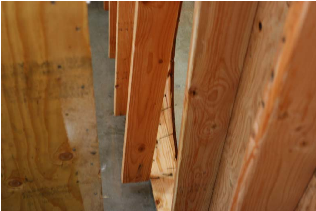
Fig. A.4: Stud to bottom plate connection failure of transverse wall
