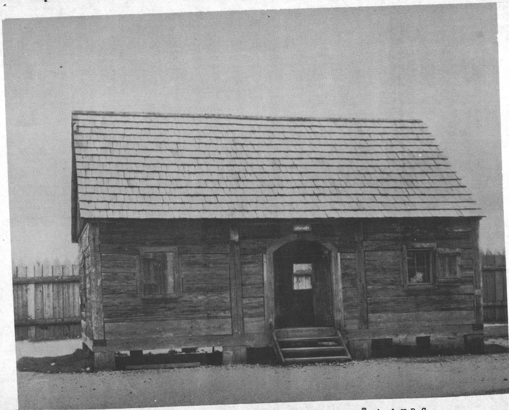
PLATE IX. Caption: Granary, Fort Nisqually, Showing Typical H.B.C. "Posts in the Sill" Construction.
