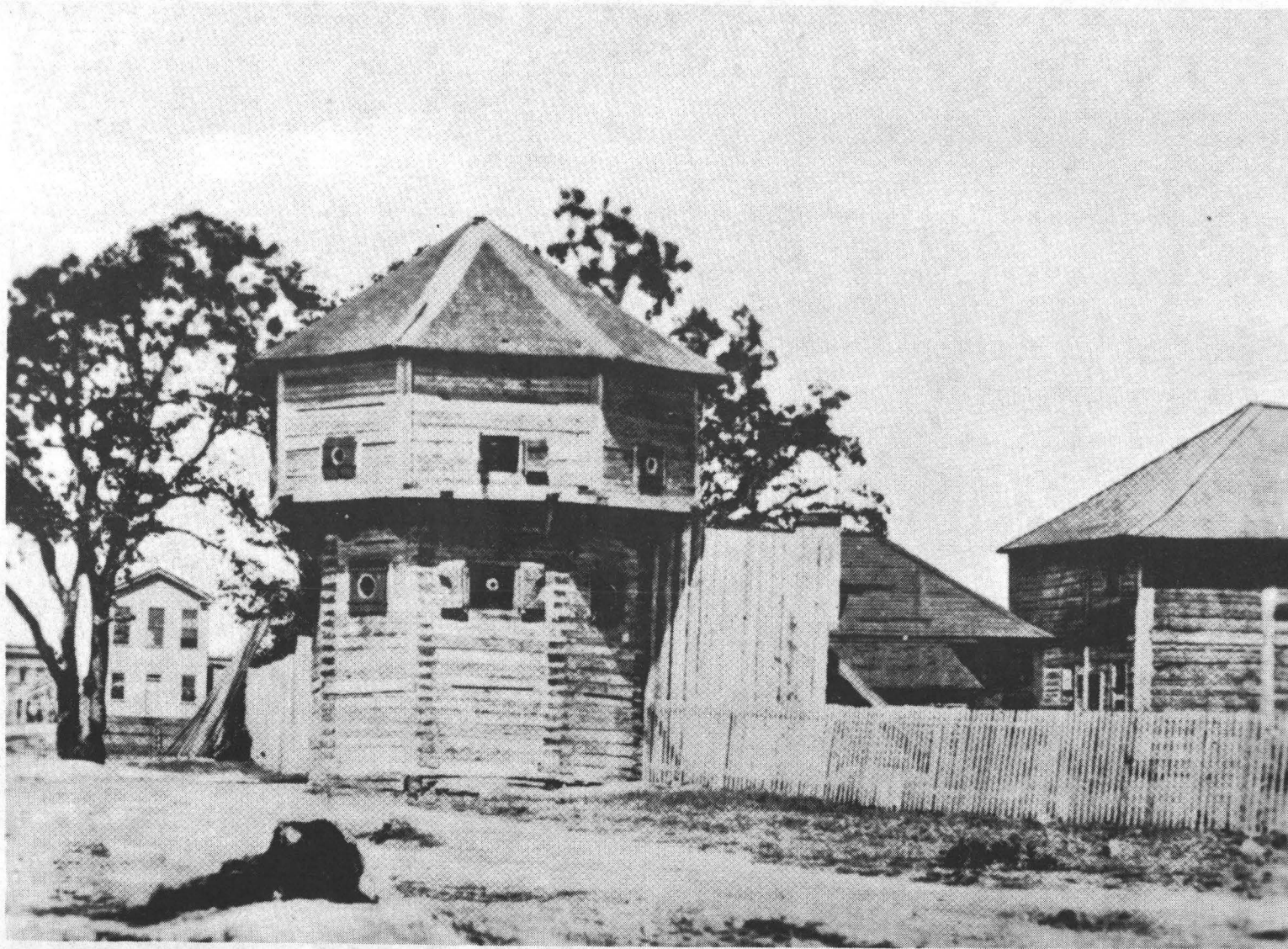
Plate VII. Caption: Bastian at Fort Victoria, Vancouver Island, Showing Typical Construction of Octagonal Cap and Gun Ports.
