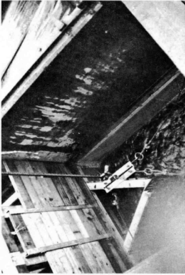
Figure 11. Upstream Adult Trap with Easily-Opened Gates, in Lowered Position.
