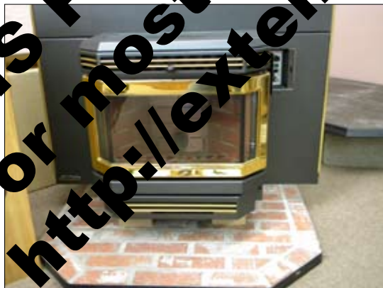
Figure 4.—Pellet stoves are more efficient than an open fireplace.
