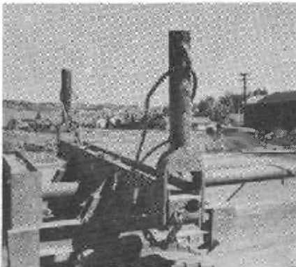
Figure 1.--Safety trip stake.
