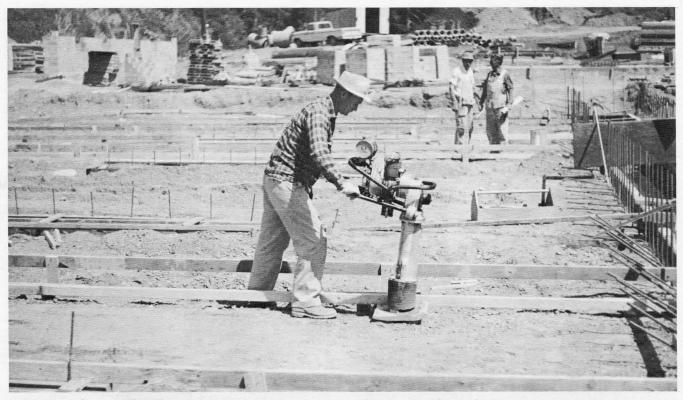
Construction began on the Fish Commission's Elk River Hatchery during the biennium. This "gadget" is compacting the soil beneath what will be the hatchery's rearing ponds.
