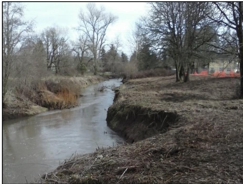
Figure 1.3- Photo of Ash Creek during LWC Restoration Project. Note the straightened channel, lack of vegetation, and incised banks.
