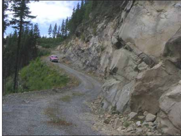
Figure 4.9. Full-bench construction ensures that no unstable fill material is placed along the outside edge of the road and that hillslopes below the road remain at their natural angle of repose.
