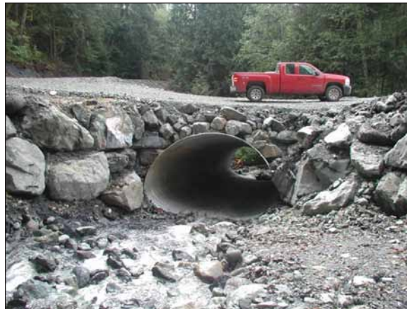
Figure 4.10. Dipped rock fills result in stable road prisms at stream crossings. Note the large-arch culvert, heavy-rock armorings, and minimal fill over the culvert.
