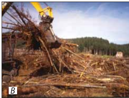
Figure 5.19. Replacement of (A) topsoil and (B) organic matter (logging slash) during rehabilitation of a temporary logging access road.
