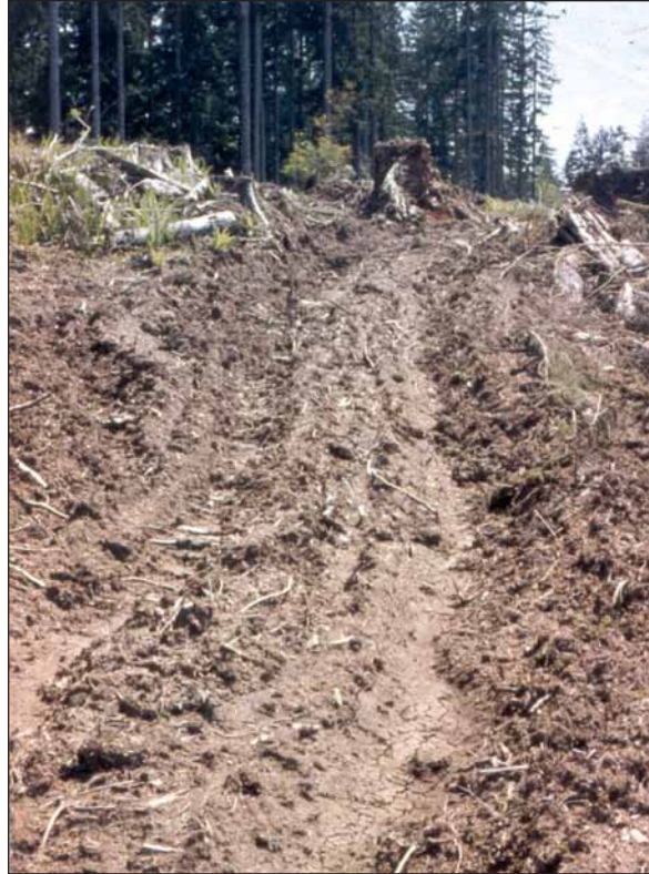
Figure 5.17. Deeply rutted Class 3 soil disturbance with the potential for erosion and movement of sediments into streams.
