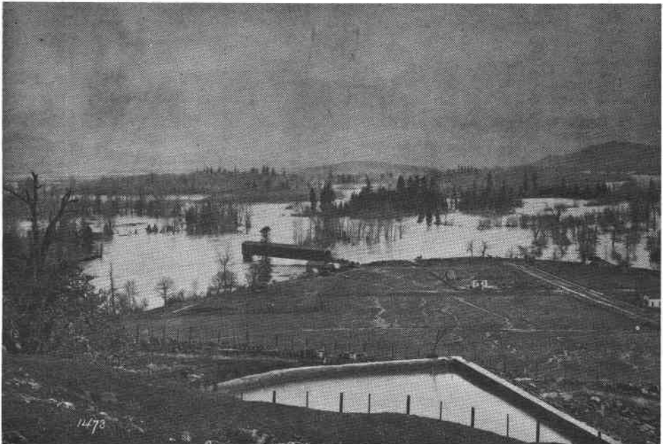
Ferry Street bridge, built in 1876 and shown in the flood of 1890, with the north approach washed away.
