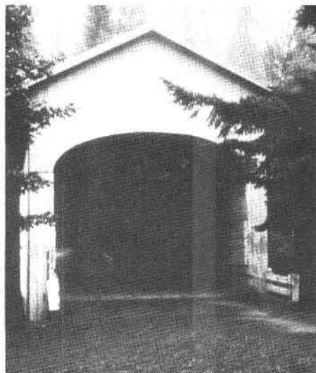
Belknap bridge no longer spans the forested banks of the McKenzie river after being swept away during the winter floods.
