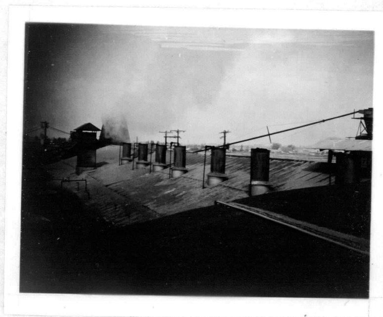
Figure 3. Vent stacks of the veneer dryer.
