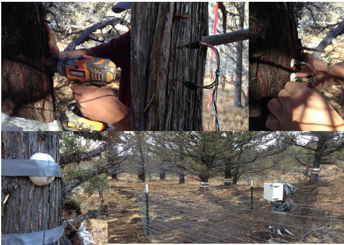
Figure A4.2. Installation of automated water use equipment in the field for the area (untreated watershed) dominated by mature juniper.
