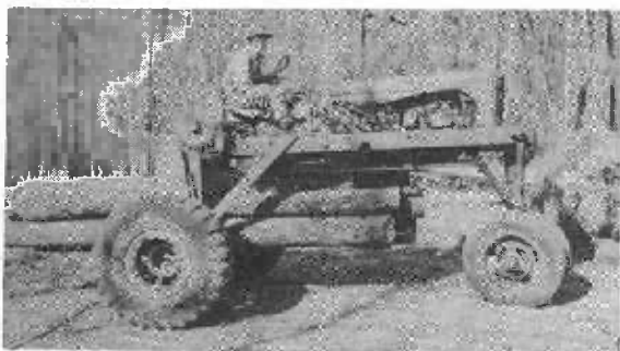
Figure 1.--Straddle tractor carrying logs.
