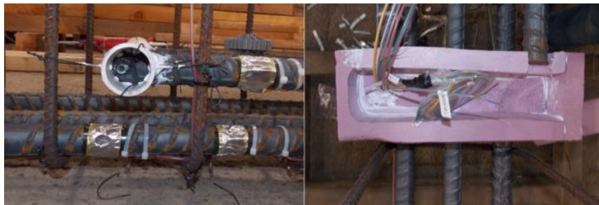
Fig. 3.10 - Cutoff bar slip sensor ports (left), and block-out box (right)
