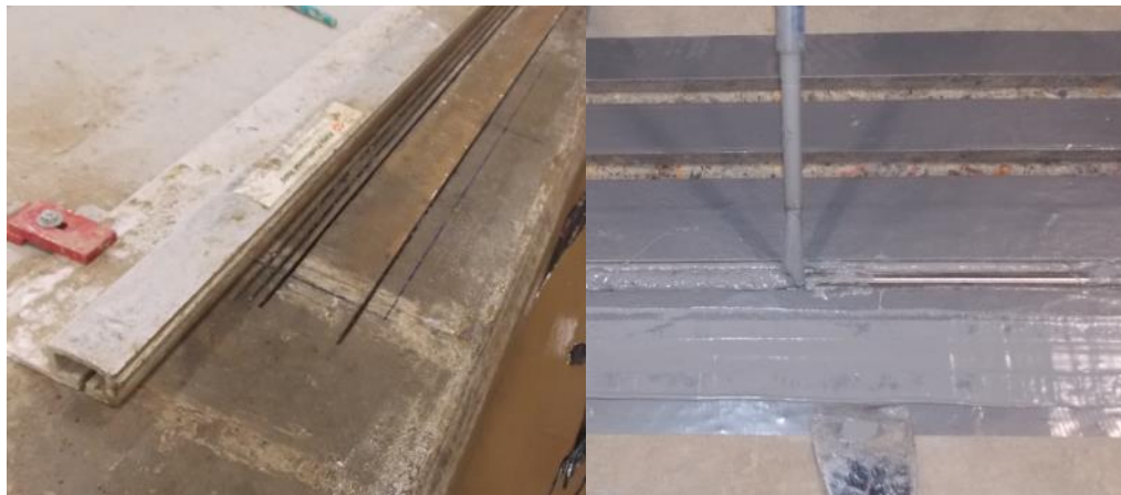
Fig. 3.14 – Saw-cutting (left) and inserting NSM bars into the concrete grooves (right)
