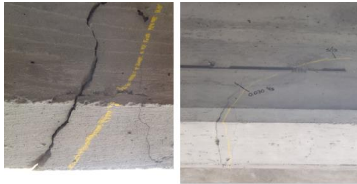
Fig. I.3 – View of haunch transition on interior girder of span 1 (right) and crack with vertical offset on interior girder of span 1(left) (ODOT 2013)
