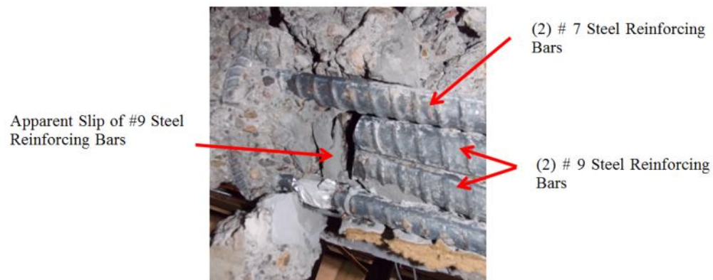
Fig. I.26 - Apparent slip of # 9 Steel Reinforcing Bars in Mosier 2
