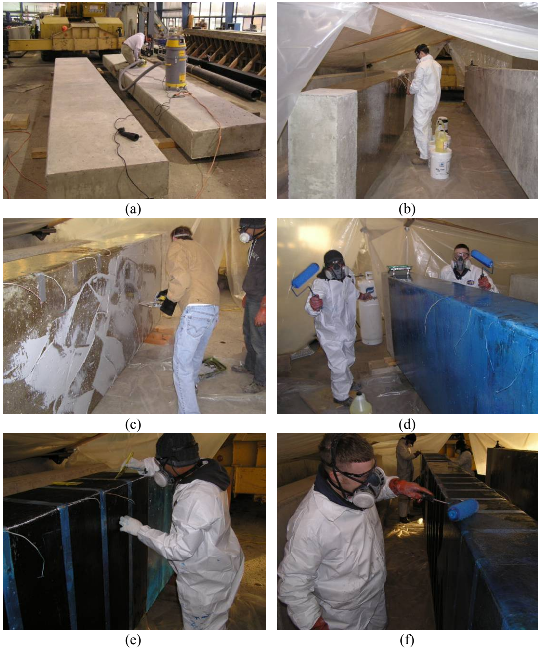
Fig. 3 – CFRP application process.
