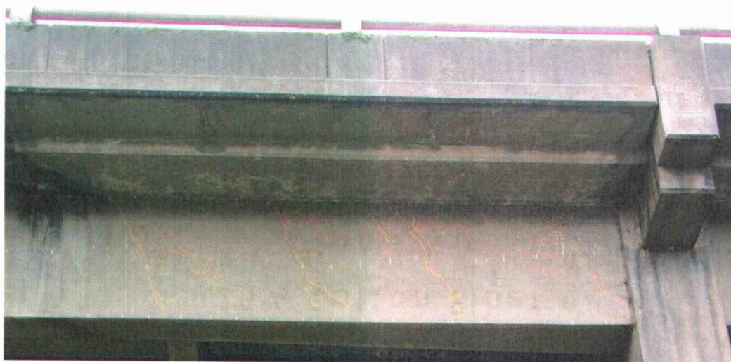
Fig. R22 – Existing cracks on the McKenzie River bridge exterior girder in span 1 near support B. The first diaphragm framing is 12.5 ft from support B centerline.
