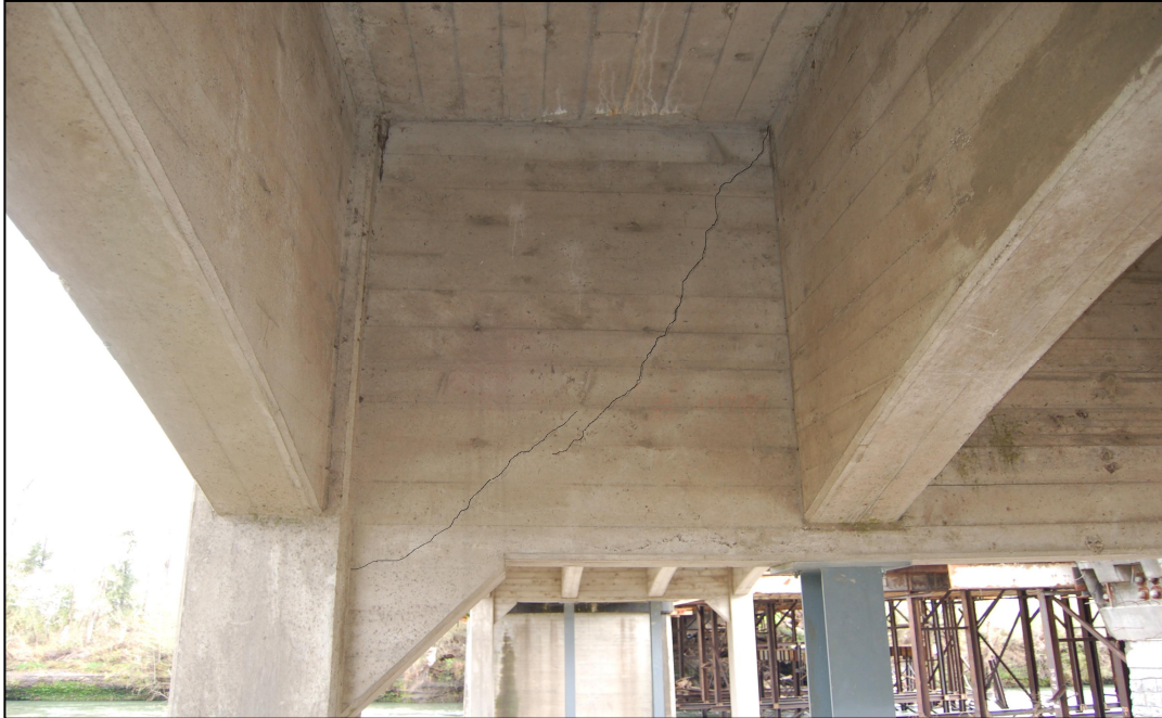
Fig.R1-Typical diagonal crack forming at column bent connection (diagonal crack highlighted).
