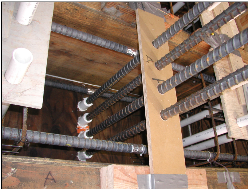
Fig. R6-Typical low confinement column cage prior to casting (no ties located in the anchorage zone).
