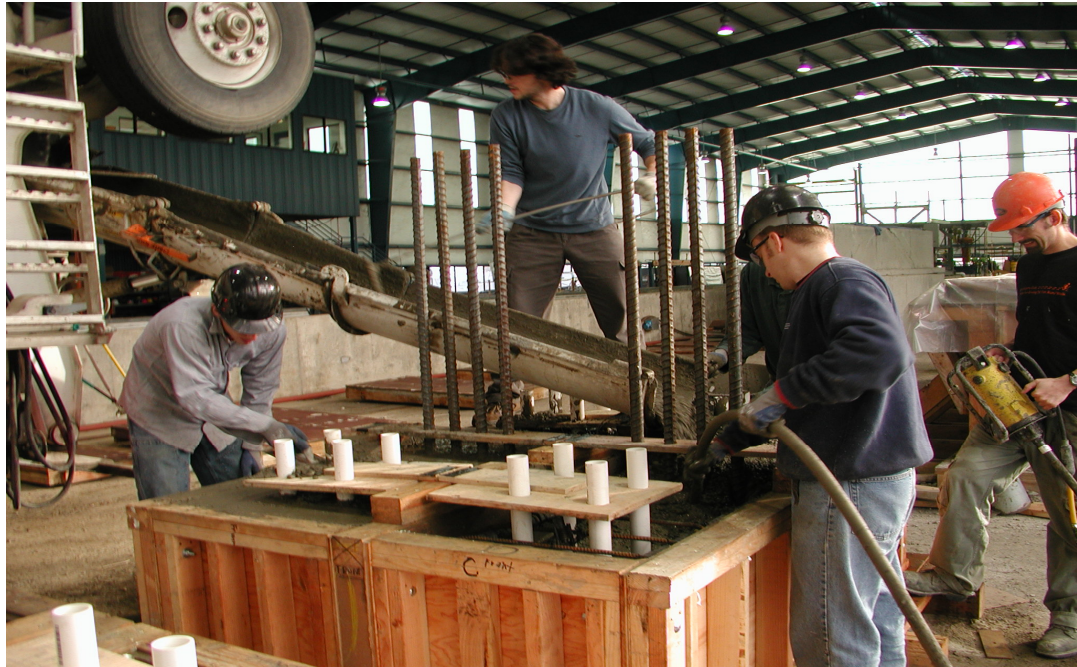
Fig. R8-Placement of concrete into formwork.
