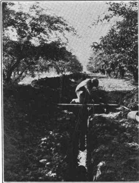
Figure 4. Boring relief well in bottom of tile trench.
