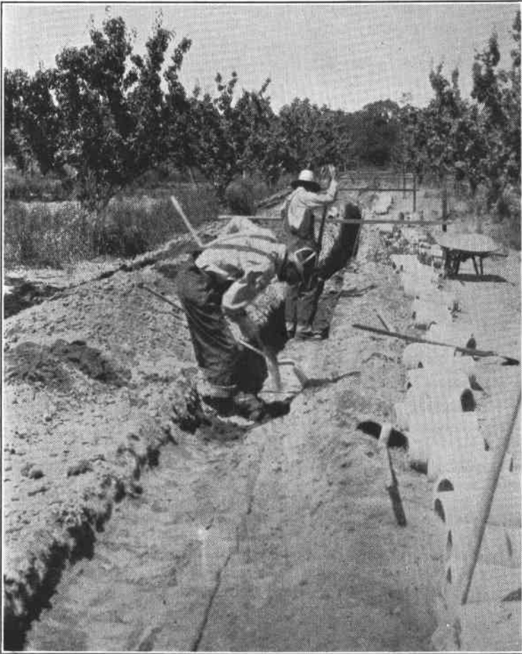
Figure 7. Excavating trench for drainage line.
