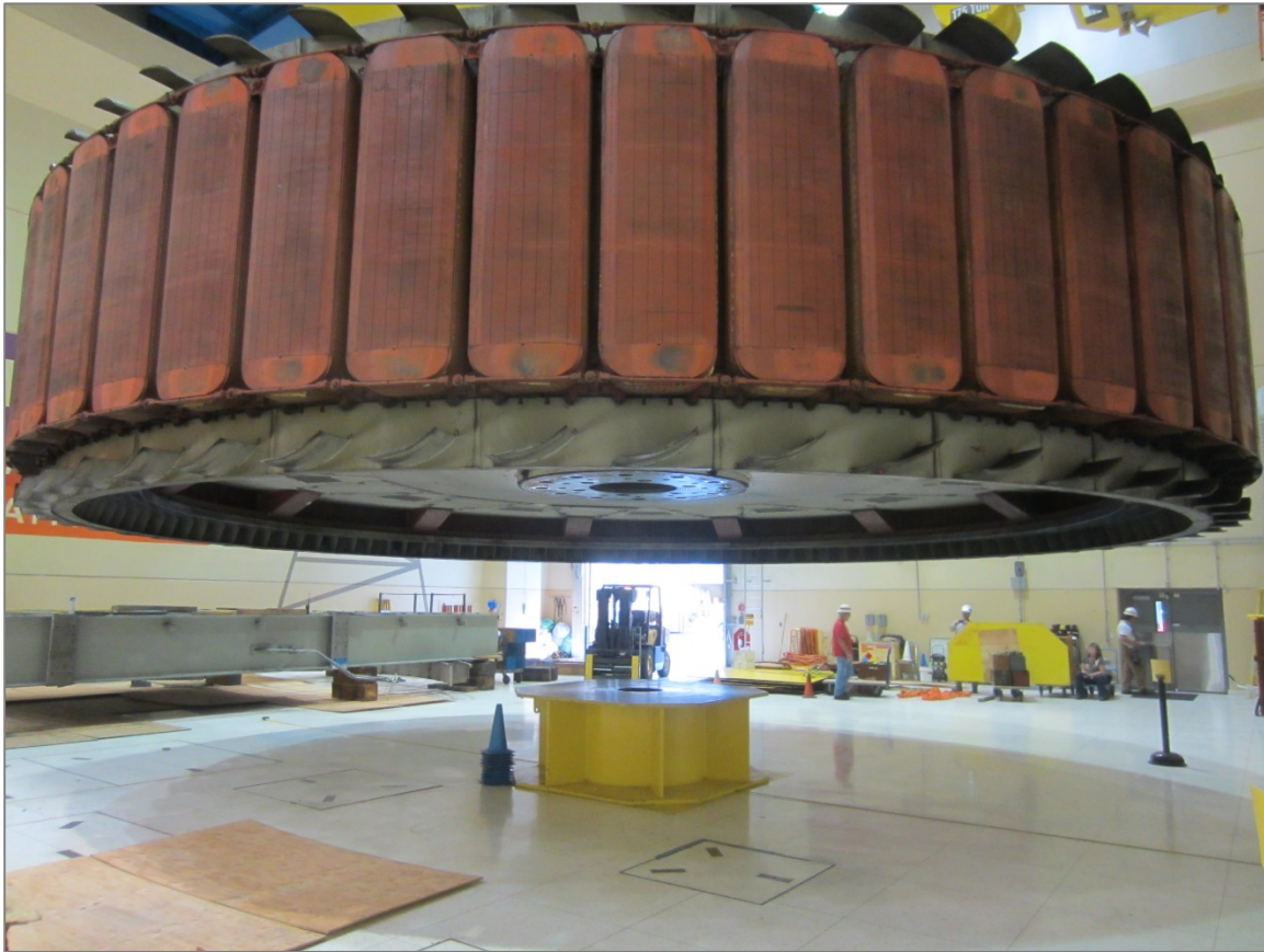
Figure 2.13: A salient pole rotor which would be connected to the runner shaft of the hydropower unit. Picture courtesy of Sean Brosig.
