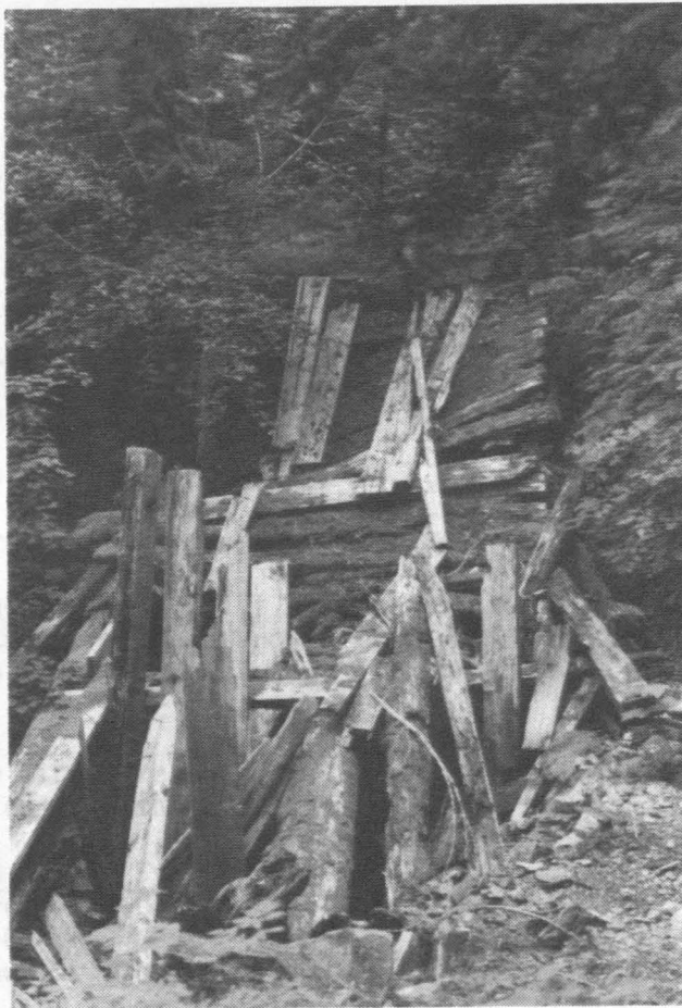
Collapsed bridge on tram road.
