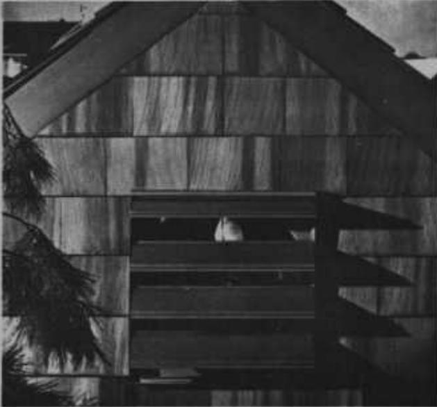
Wall-mounted attic fan is installed on end wall or gable of attic. These units fit between studs, come in sizes from 600 to 2100 CFM (rated at 0.03 inch static pressure) with 1/15 to 1/4 hp slow-speed (1025-1550 RPM) motors. Self-closing louvers need no insect screen; fixed louvers should have insect screen.
