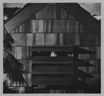
Wall-mounted attic fan is installed on end wall or gable of attic. These units fit between studs, come in sizes from 600 to 2100 CFM (rated at 0.03 inch static pressure) with 1/15 to 1/4 hp slow-speed (1025-1550 RPM) motors. Self-closing louvers need no insect screen; fixed louvers should have insect screen.
