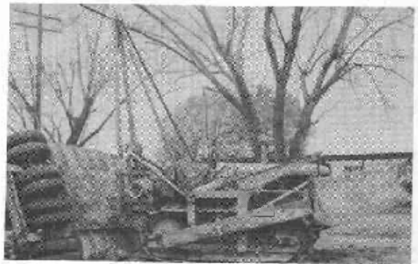
Figure 2.--Boom attached to tractor winch bracket.
