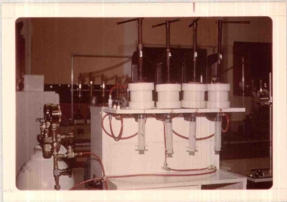
Figure 1. Interstitial water sampler.
