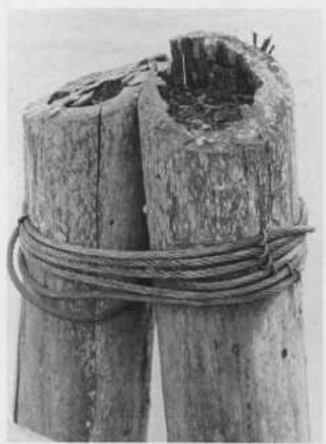
*This beam end shows preservative penetration—but nothing will protect its interior from moisture . . . there was no protection, either, for the sawed-off ends of these piles. . . .*
