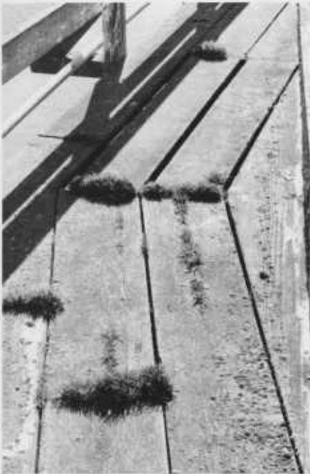
*Water condenses on a window frame . . . joined surfaces on this deck have absorbed moisture (the grass tells it all!). . . .*
