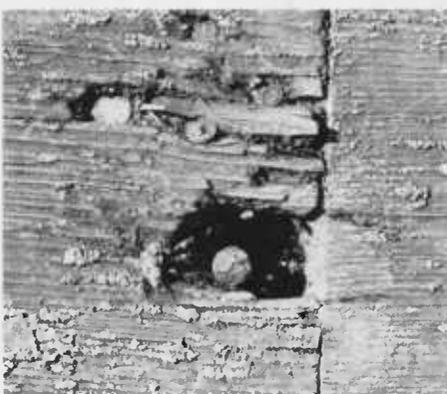
*Seasoning checks trap water . . . bolt and nail holes absorb it, too. . . .*
