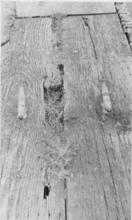
*Decay problems can also arise in pressure-treated wood—decay within seasoning checks that open past the protective shell; decay resulting from inadequate treatment. For information on what to do about this, see the slide tape, Improving the Performance of Wood in Waterfront Structures (page 8).*
