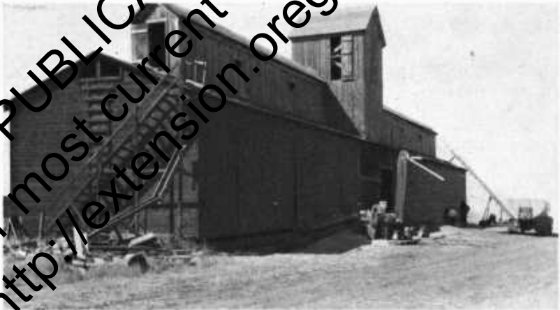
Figure 9. Closing doors and screening windows and other openings in grain-storage buildings will eliminate most contamination by birds.
